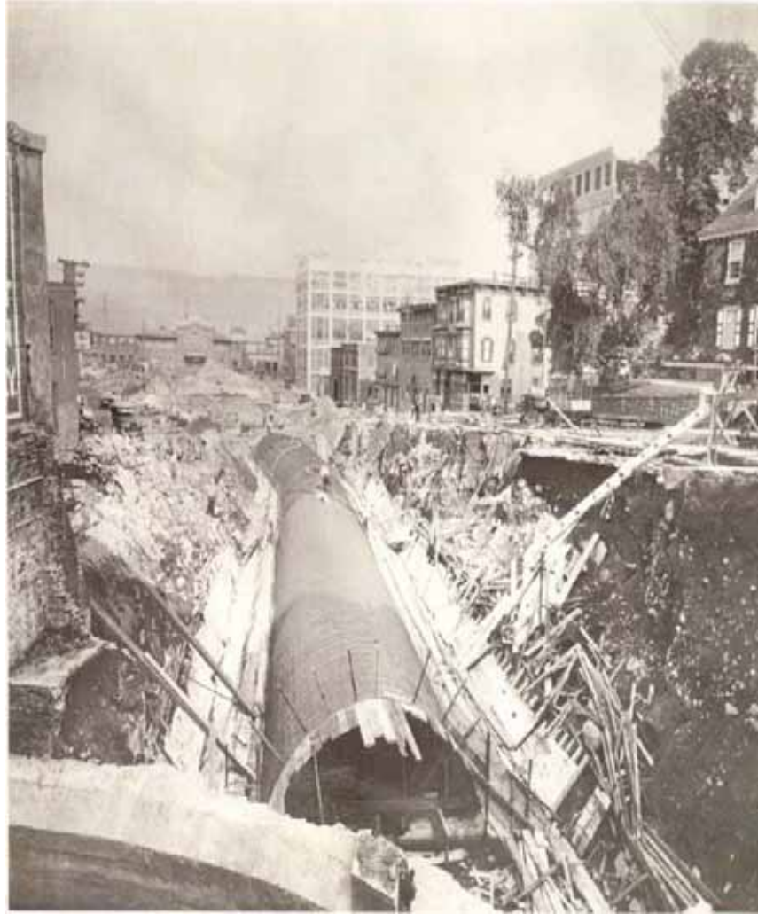
Photograph 229. Structure 532, Sawmill River flume/culvert under Larkin Square and North Broadway, constructed in 1946 (Historic photograph).
